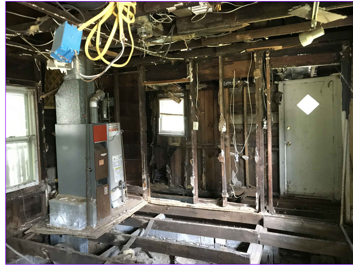
5 EXISTING INTERIOR VIEW (FACING REAR) NOT TO SCALE
